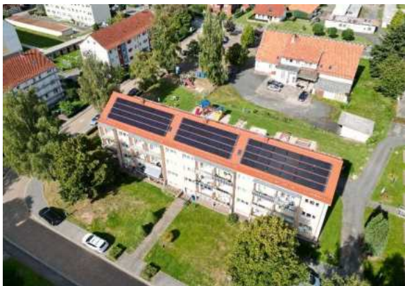
Photovoltaik-Thermie-Anlage in Arenshausen
